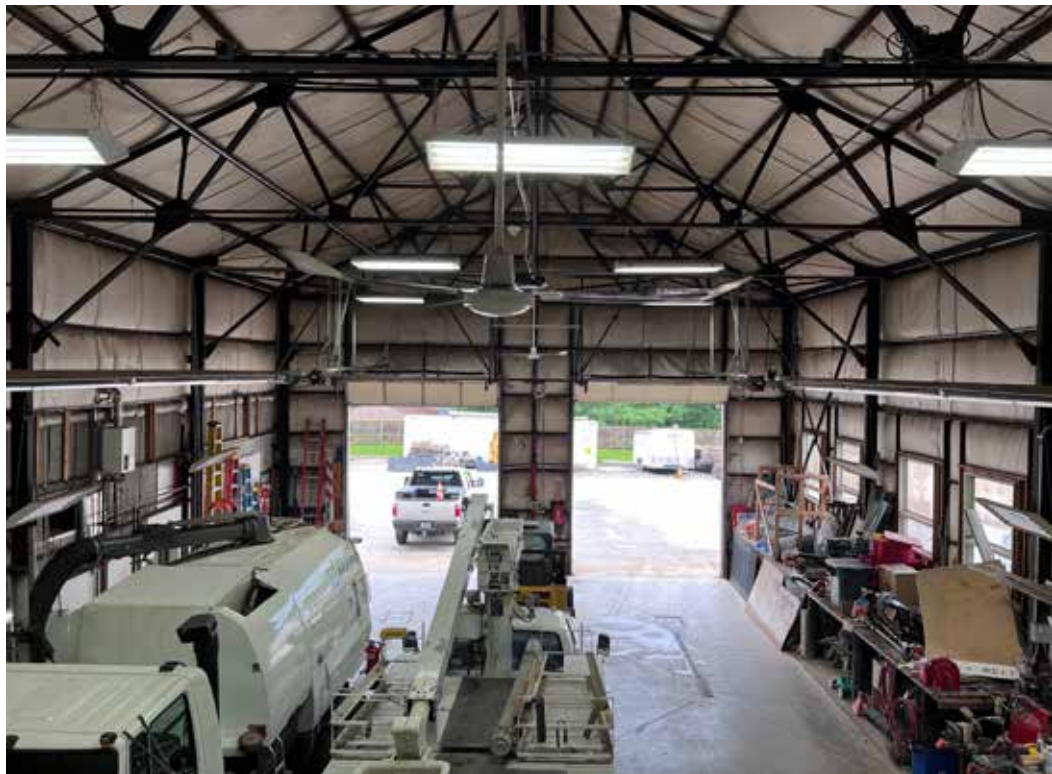
Truck bay without exhaust ventilation system
