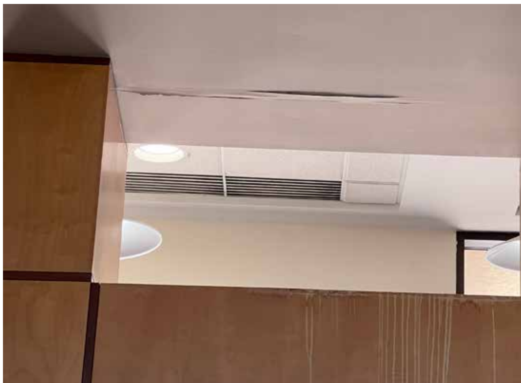
Interior ceiling and finish damage due to roof leak
