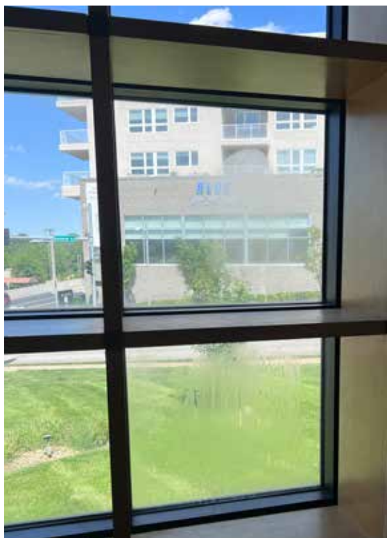
Failing glazing units
