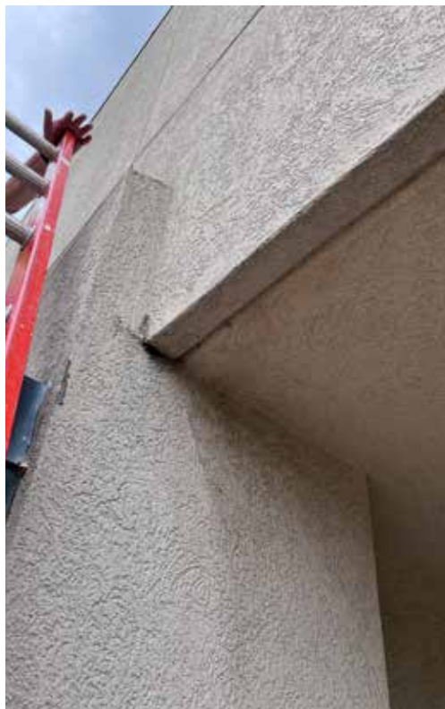
Damaged EIFS cladding
