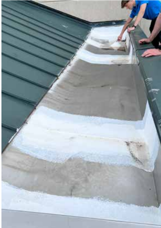
Leaking roof gutter
