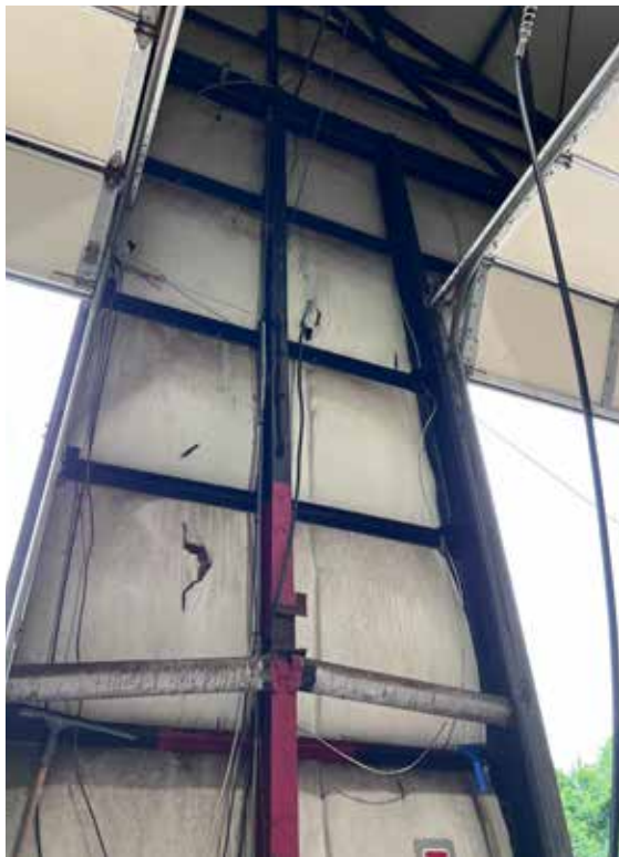
Damaged insulation on wall panels
