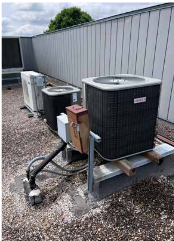
Mechanical units on original ballasted roof
